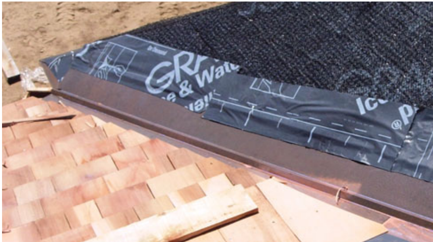
Figure 4. The author culls shingles more than 10 inches wide from the bundle and uses them to make one-piece valley cuts.
