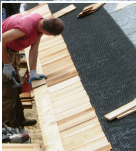
Figure 7. To start the first course, the crew nails a guide strip to a chalk line snapped at the 1½-inch overhang (above). Fence boards ripped to the exposure width guide the successive courses (right).
